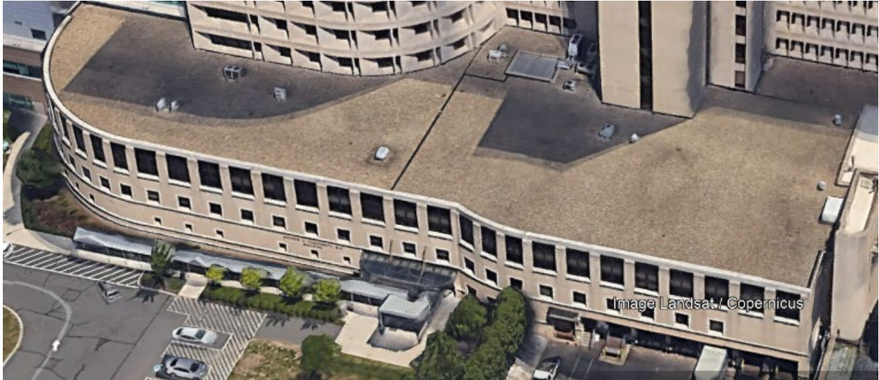
BUILDING F (CANZONETTI BUILDING) ROOF
