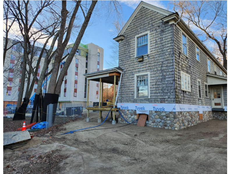
4 Gilbert Road - House Relocation
