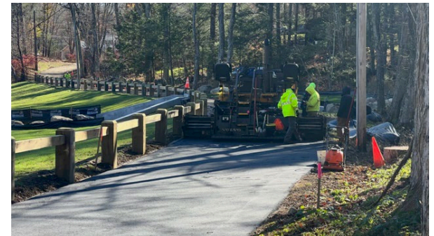
New Roadway being installed
