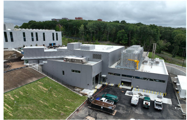
SUP View Looking South
