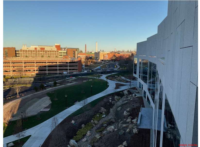
North Elevation Looking East
