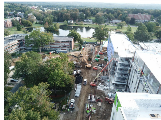
Installation of new utilities in Gilbert Road
