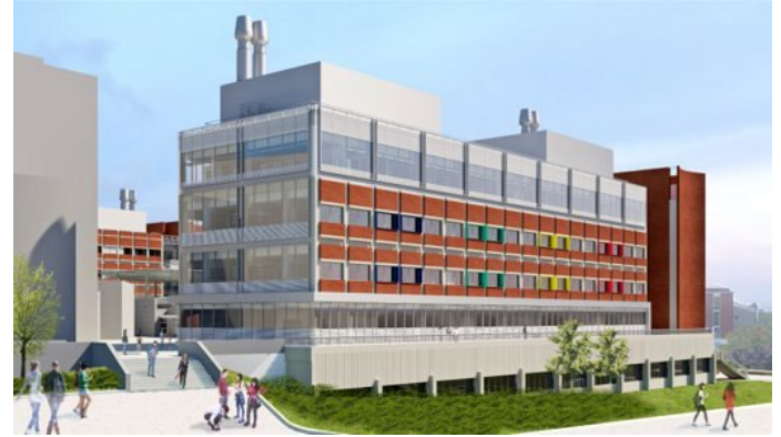
View of 4 th Floor North Wing Addition from North Eagleville Rd
