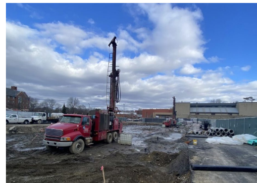
Installation of geothermal system, S Lot 7
